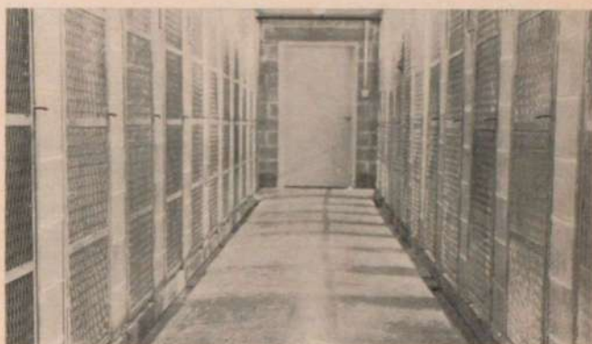
Pic. #3—with drain troughs
